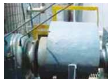
Petrochemical Complex, Mexico
